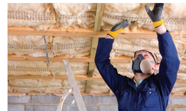
19. R6.0 Top Storey Trussed Roof Ceiling Insulation
