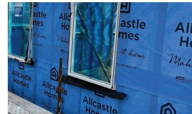
20 & 21. Heavy Duty Roof & Wall Sarking
